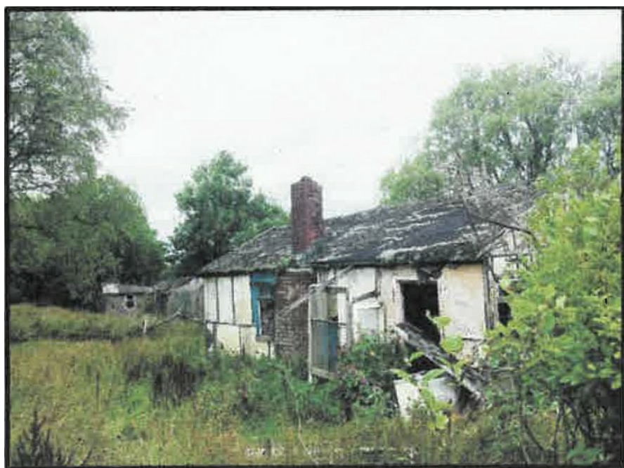
Derelict bungalow, Chinatown
