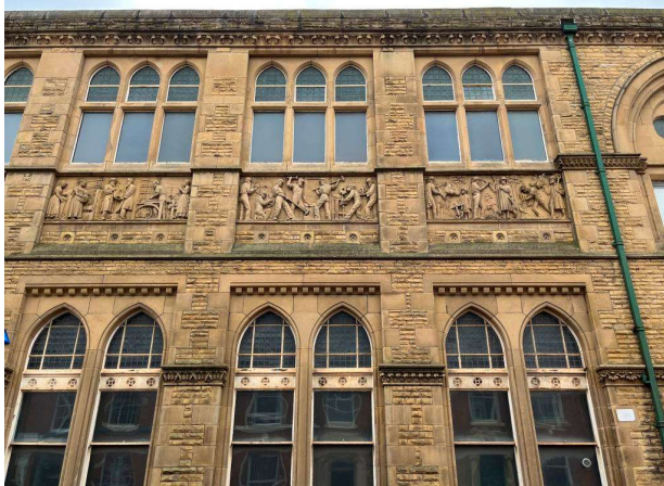
Sculpted panels on the front (top) and side of the Museum and Art Gallery building
